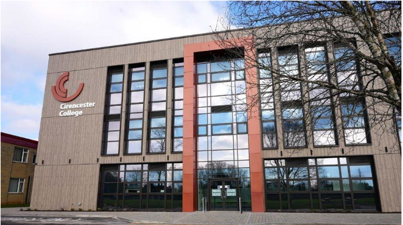
New T Level Building, including T Level Construction
